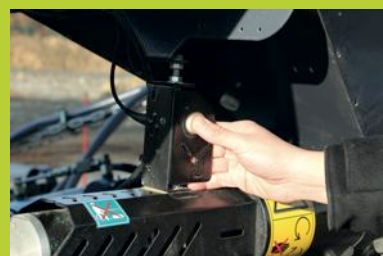
Calibration test button Placed near the distribution
